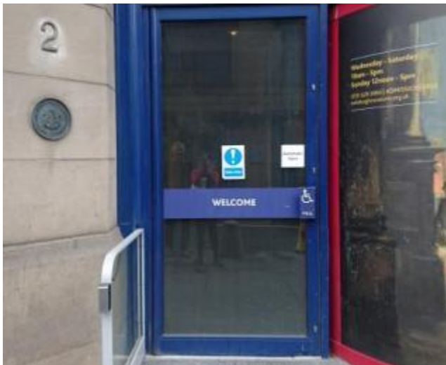
Front door from outside
